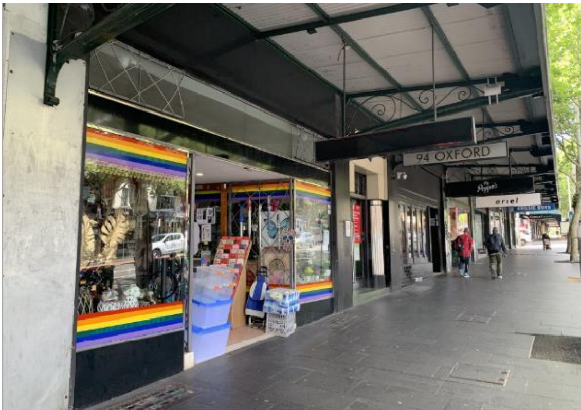
Figure 13: Shopfronts of Group 2
