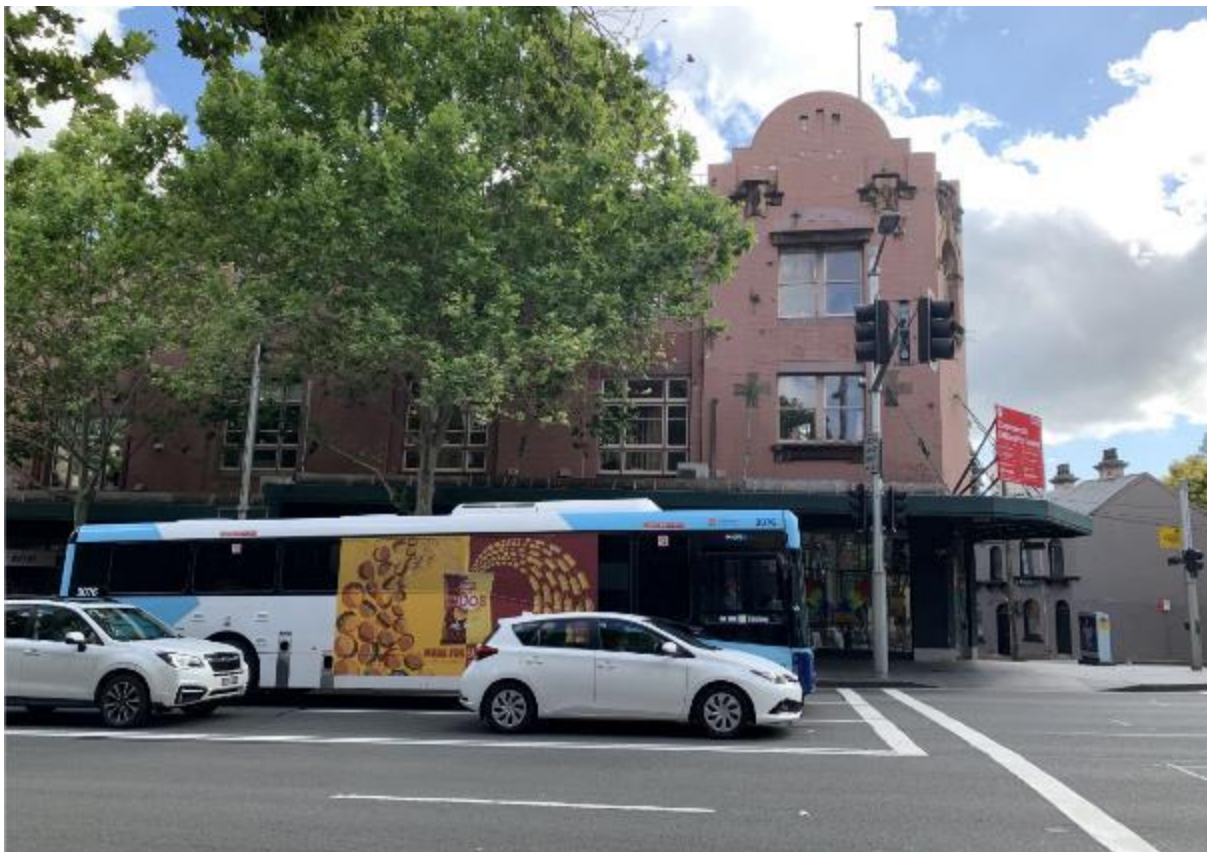
Figure 11: Group 2 as viewed from the corner of Oxford Street and Palmer Street
