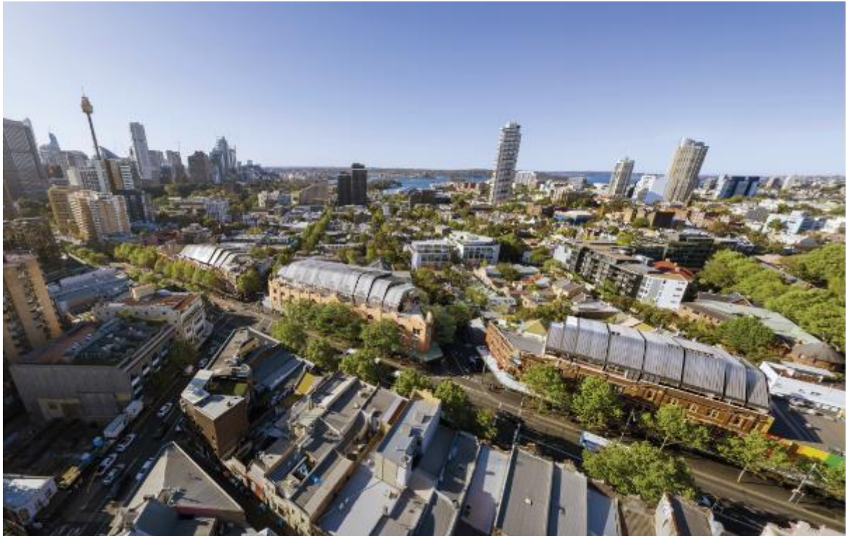
Figure 27: An aerial view of Group 1, Group 2 and Group 3 viewed from the south-west (Note: Group 3 is not the subject of this report)
