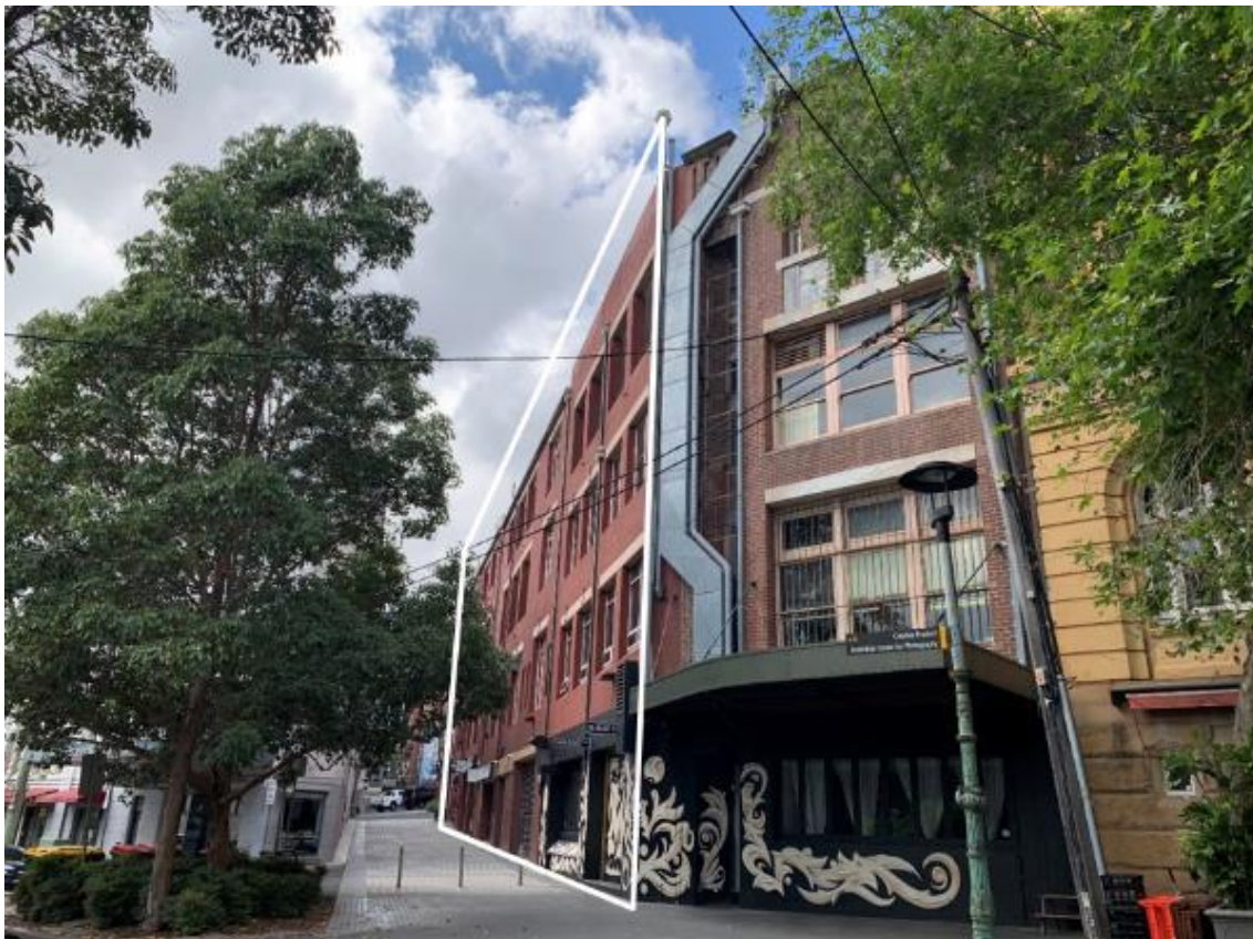
Figure 4: The site looking south east along Foley Street from Oxford Square
