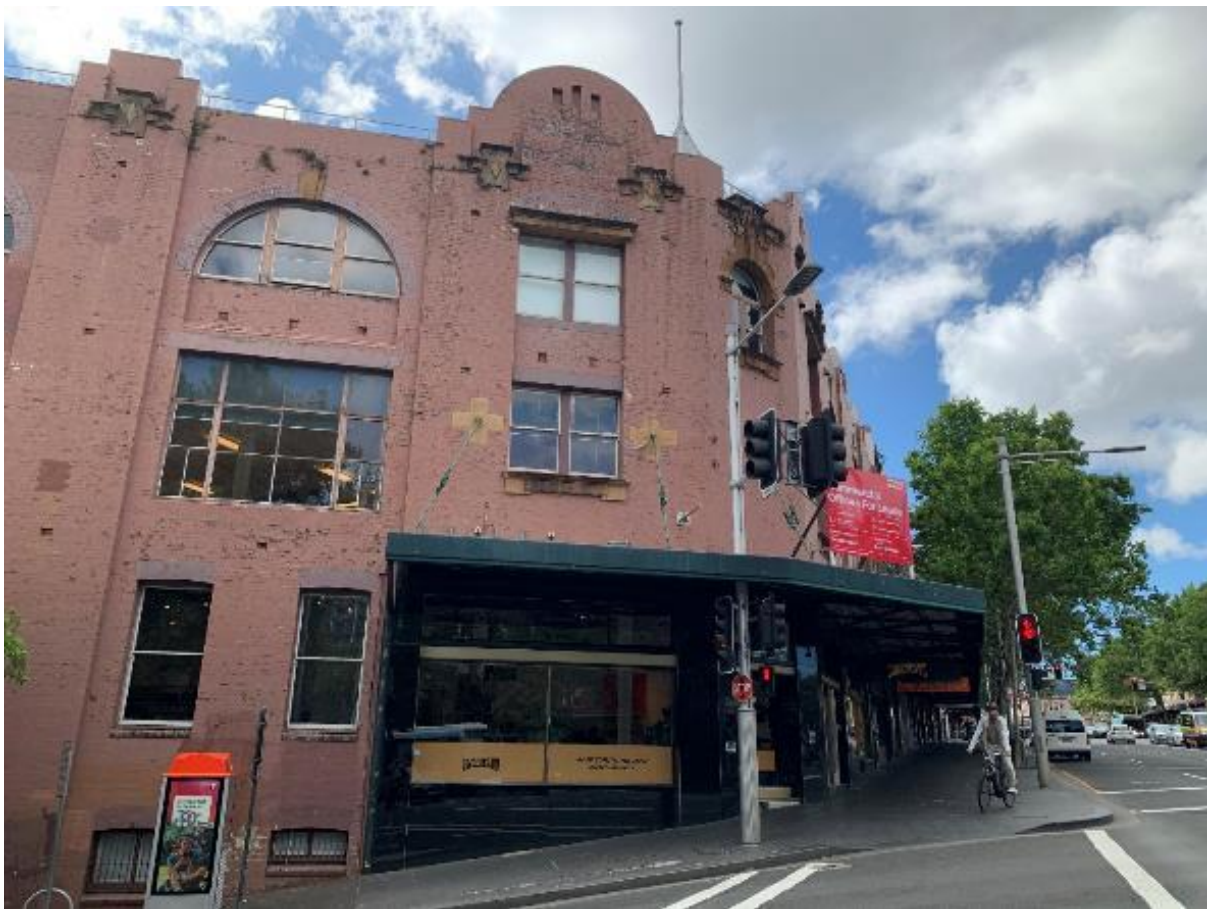
Figure 9: Group 2 as viewed from Crown Street
