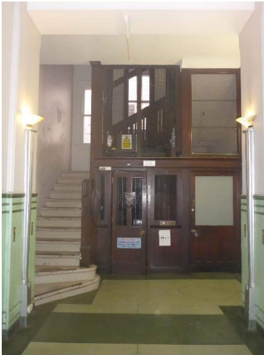
Figure 18: Original lift shaft and stairs of Group 2
