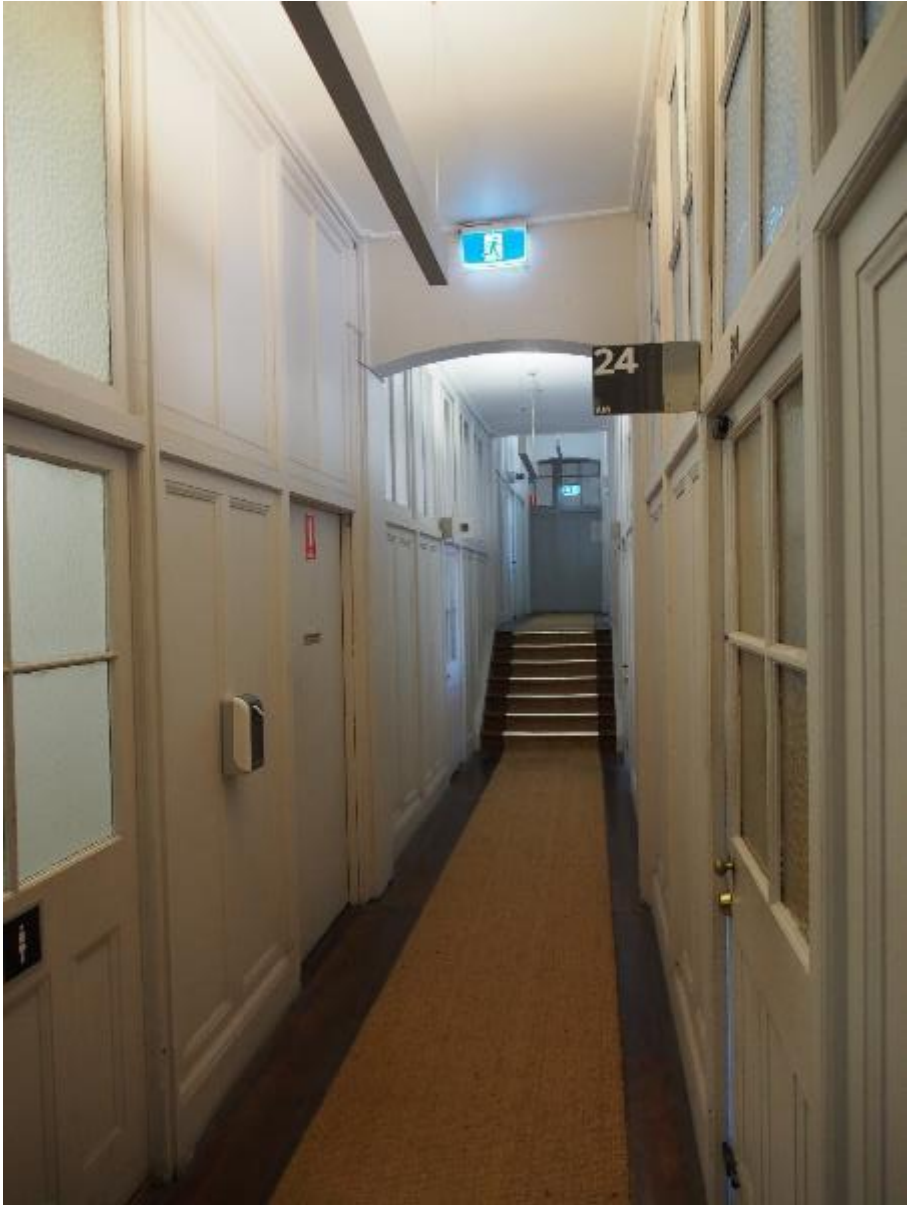
Figure 20: Hallway of Group 2 (Level 2)
