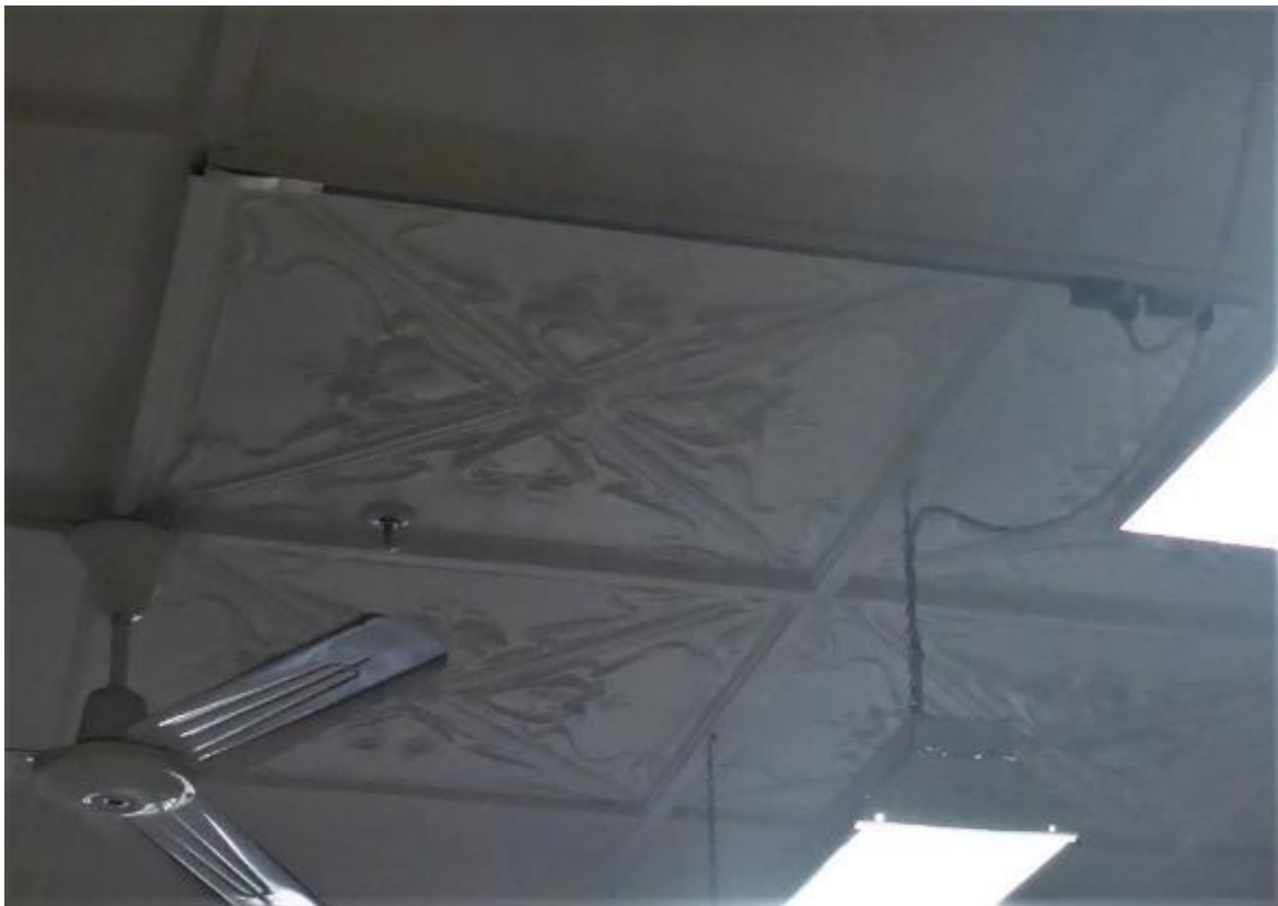
Figure 22: Original ceilings within Group 2
