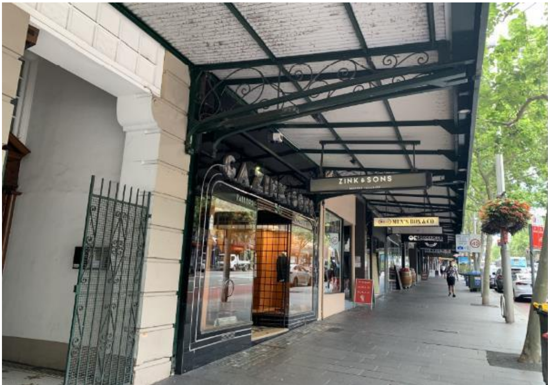
Figure 6: Group 1 shopfronts along Oxford Street and 56 Oxford Street (GA Zink & Sons), which is not part of the DA, shown in the foreground
